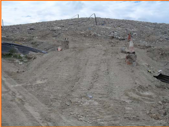
Uncapped waste, with gas extraction pipes seen at top
