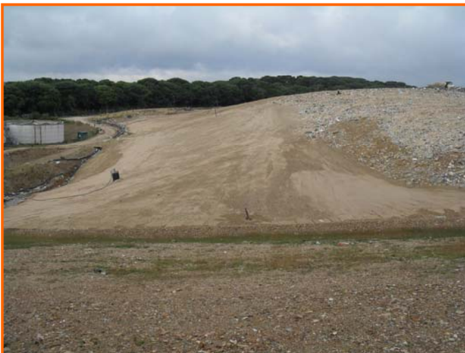
Waste capped with regulated material on left section
